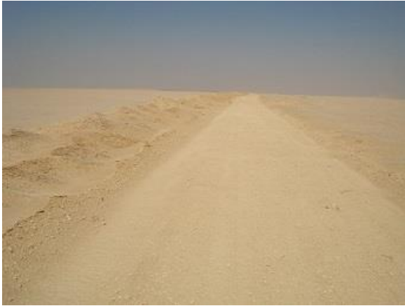
Figure 5-11: Provisional gravel road at WP 6_2 (upper layer of 30 cm removed)
