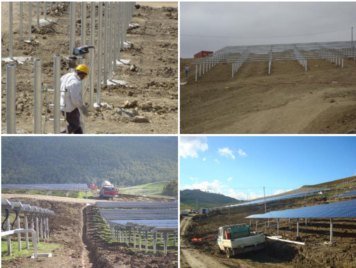
Figure 3-11: Fixed mounting structures assembly (source: Lahmeyer, Cammarata PV Plant in Sicily)
