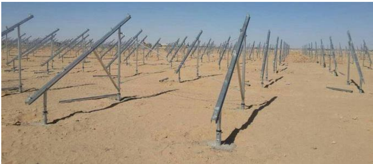
Figure 8: Typical 'Mounting Structure' erected on site
