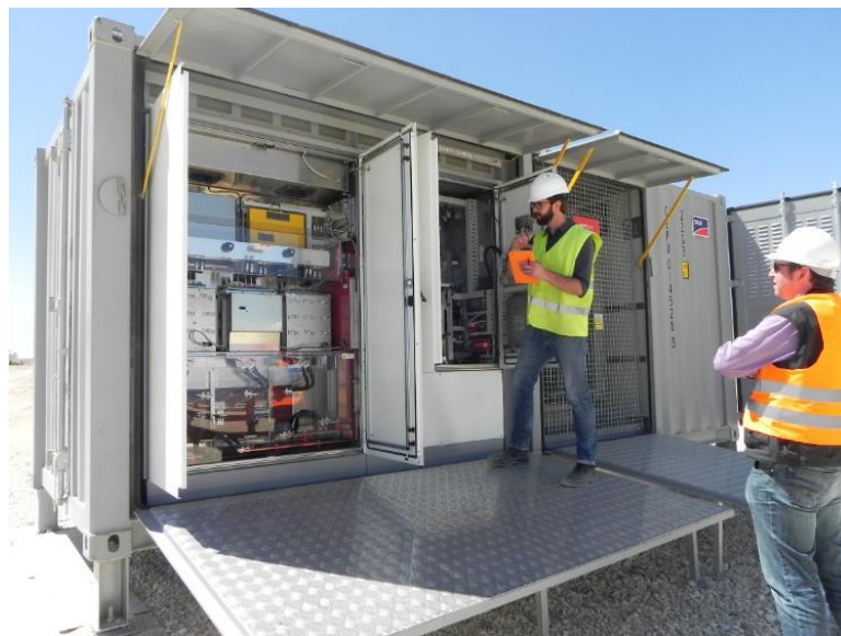
Figure 3-14: 2 x 1,010 kW PV switchgear in Jordan
