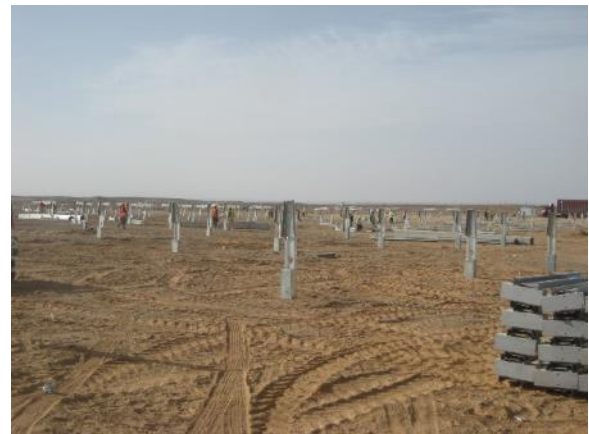
Figure 3-6: Mounting structure concrete foundation (Al- Ward Al Joury PV Plant –Jordan)
