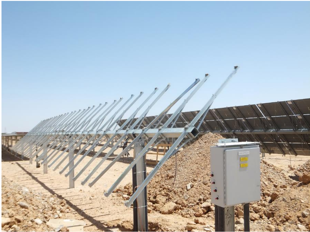
Figure 3-2: Typical 'Mounting Structure' erected on site (source: Lahmeyer, Shams PV plant in Jordan)
