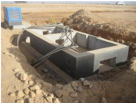
Figure 3-8: Inverter foundation example (Source: Lahmeyer, Falcon PV plant in Jordan)
