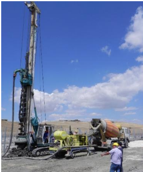
Figure 3-7: Depth mounting structure foundation construction (source: Lahmeyer, Mussomeli PV plant in Sicily)
