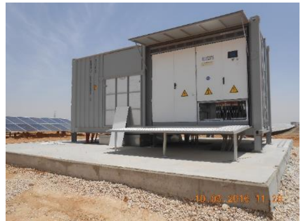
Figure 3-8: Inverter foundation example (Source: Lahmeyer, Falcon PV plant in Jordan)
