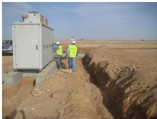
Figure 3-10: Trench cable leading cables to/from inverter (Source: Lahmeyer, Shams PV Plant in Jordan)
