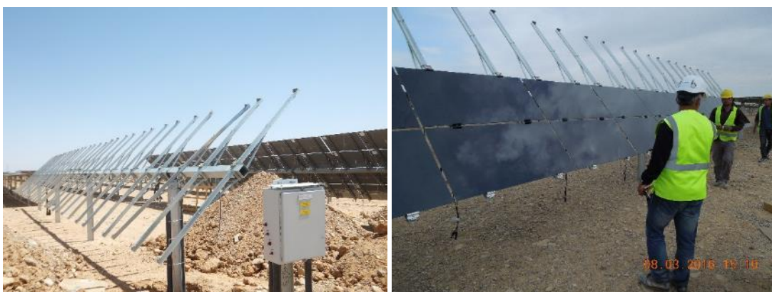
Figure 3-13: Single axis tracker mounting structure (source: Lahmeyer, Shams PV plant in Jordan)
