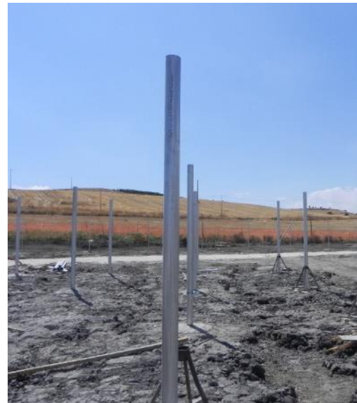
Figure 3-7: Depth mounting structure foundation construction (source: Lahmeyer, Mussomeli PV plant in Sicily)
